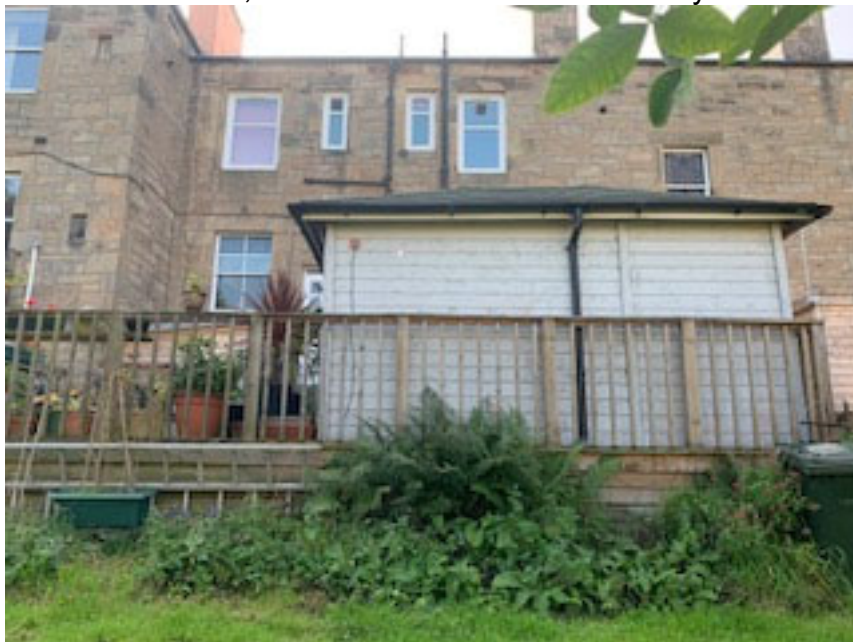
No1 – Next Door, deck and summerhouse 7 Ladysmith Rd
