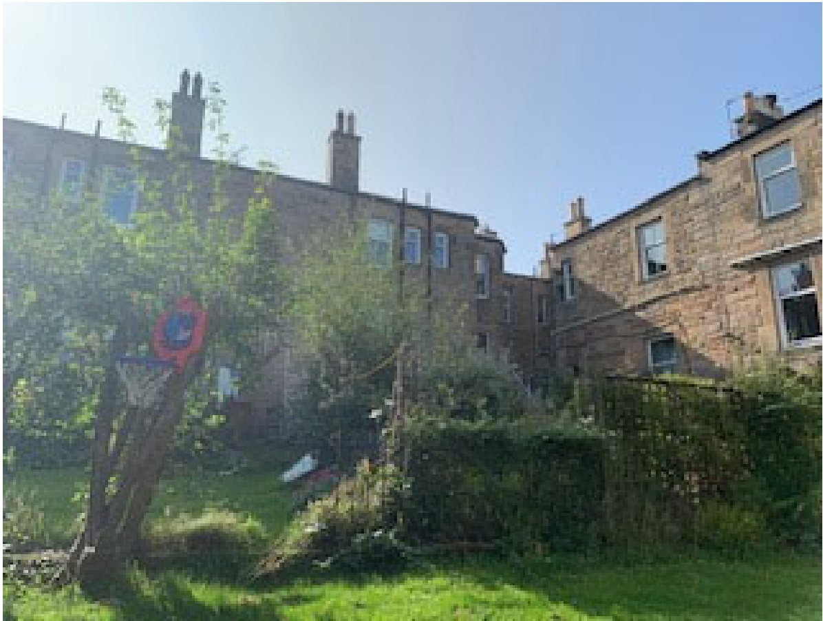
No7 View of our Structure from communal garden (can't see it!)
