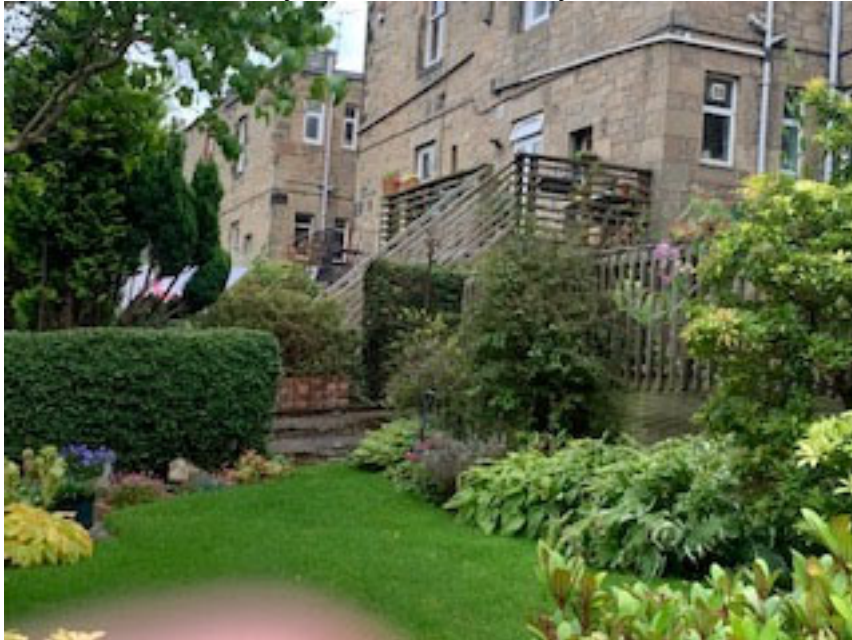
No3 Decked balcony with stairs 13 Ladysmith Rd
